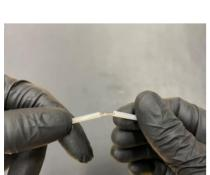
4. Snap the buffer tube to expose the inner fibers. Clean if necessary.
